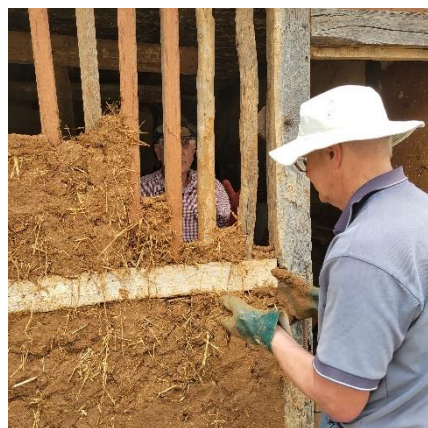
Pugging is a two-person job!
