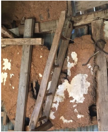
Pug walls in the cottage, showing remnants of limewash.
