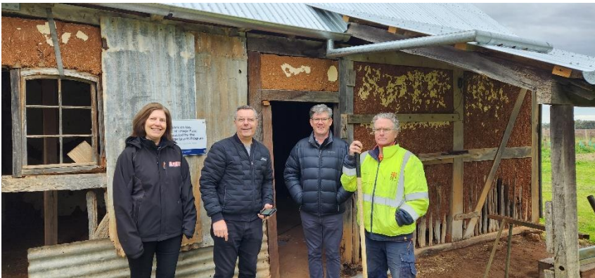
Andy Grope took this photo of Catherine Baldwin with Michael Queale (Heritage SA), Sam Hosking (Barossa Council Heritage Advisor) and Andrew Steinkopf (Heritage Builder) as they met onsite to discuss options for the footings.
