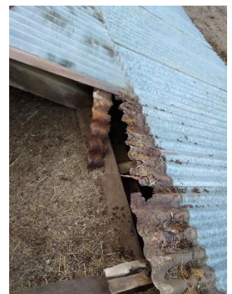
Straw is packed under the iron roof
