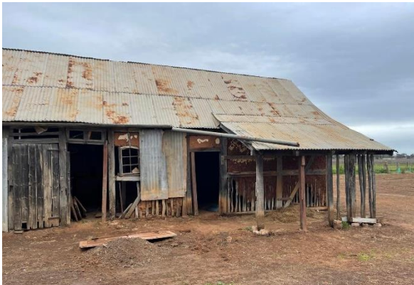
The rusted old iron roof has its own beauty.
